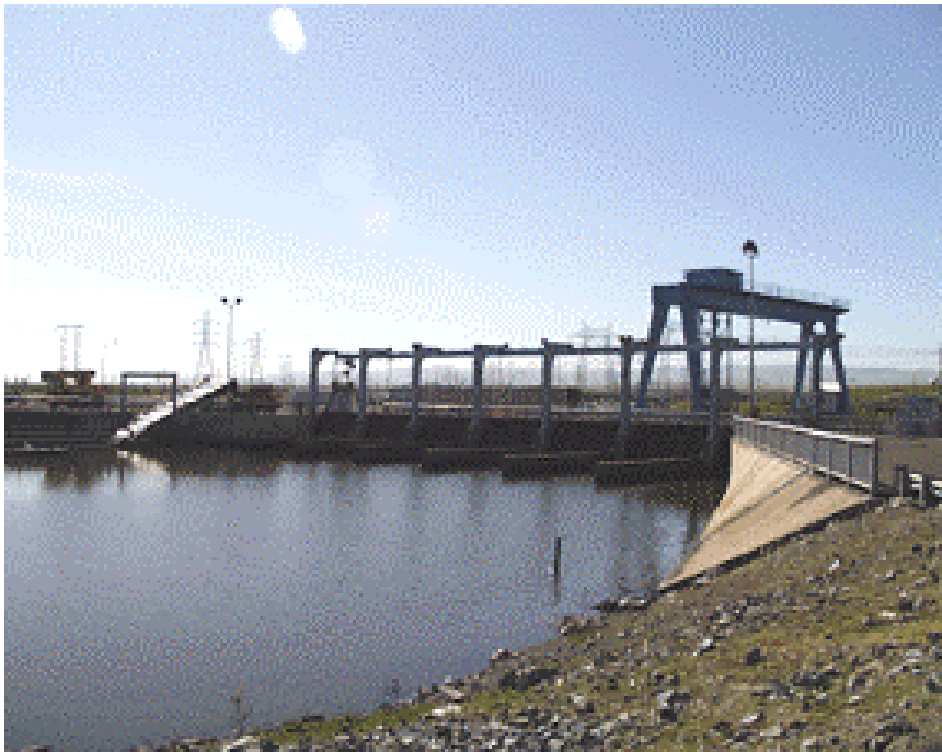
Photograph J-4. View of the Entrance to the Skinner Fish Facility Primary Louver Channels (Source: California Department of Water Resources; Photograph by Steve Foss, California Department of Fish and Game.)
