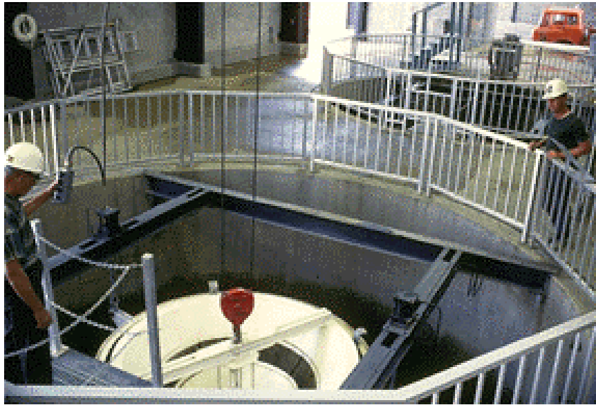
Photograph J-7. View of the Skinner Fish Facility Holding Tanks and Bucket A bucket is lowered into a holding tank to capture fish for counting. (Source: California Department of Water Resources.)
